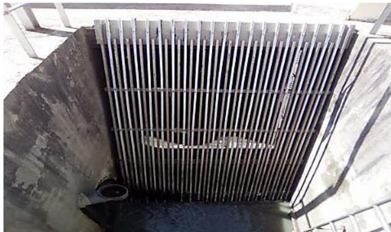
Figure 8. degraillge grossier (ONA,2022)
