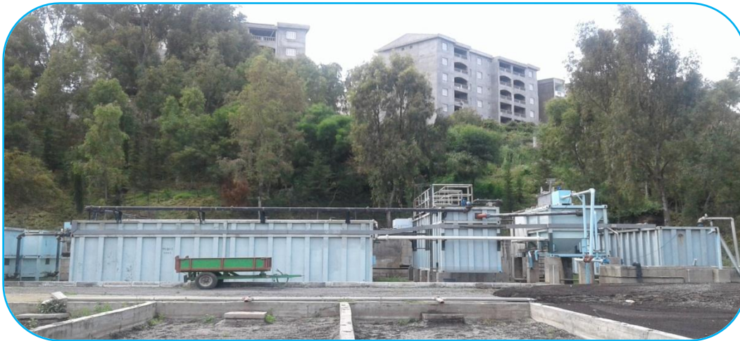
Figure 3 : ancienne station monobloc
