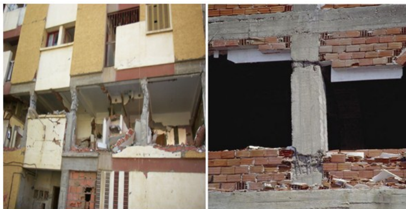
FIGURE 2.14 – cisaillement des poteaux courts
