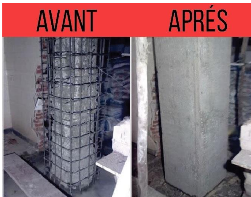
Figure 84 : La technique du chemisage. (Source : https://www.startpage.com/sp/search )
