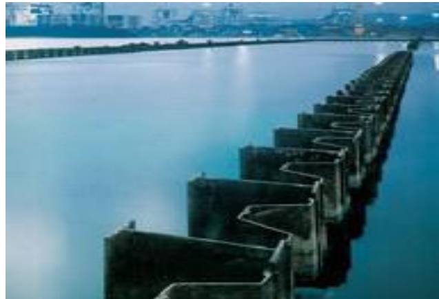
Figure 2.1. Rideaux mixtes HZ/AZ(Arcelor Mittal, 2013)
