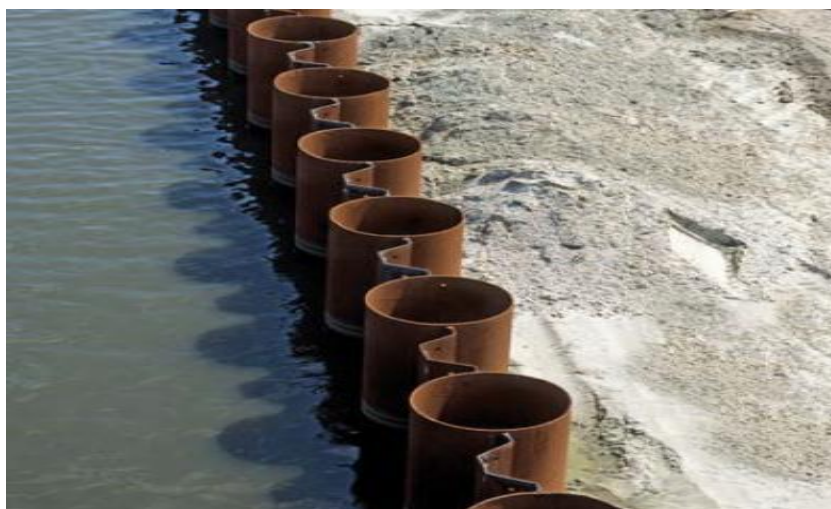
Figure 2.2. Rideaux mixtes tubes ou caissons (Ecluse, Evergem, Belgique) (ArcelorMittal, 2021) Source: ArcelorMittal
