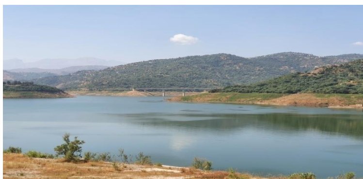
Figure 1: Photo du barrage TAKSEBT
