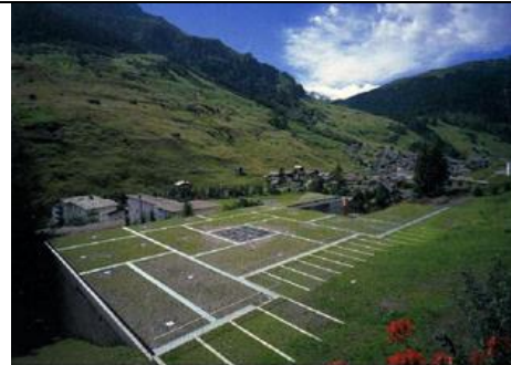
fig165 : Toiture des Thermes de Vals, source: http://amchdesign.wordpress.com/2012/02/06/Thermes-de-Vals-Zumthor/
