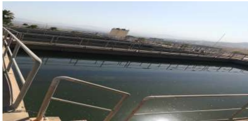
Figure III.14: Filtres AQUAZUR V
