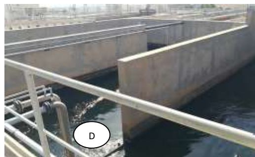
Figure III.9: Injection de Al_2(SO_4)_3
