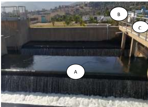
Figure III.4: Chambre de dissipation
