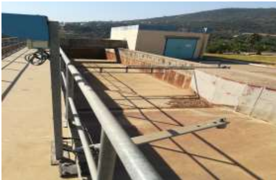
Figure III.11: Canal Parshall
