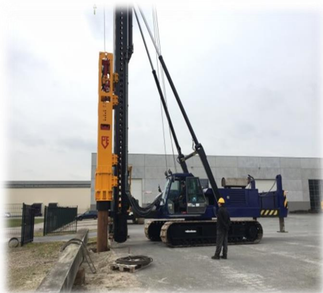
Figure 14 : Mât de battage PVE 50PR
