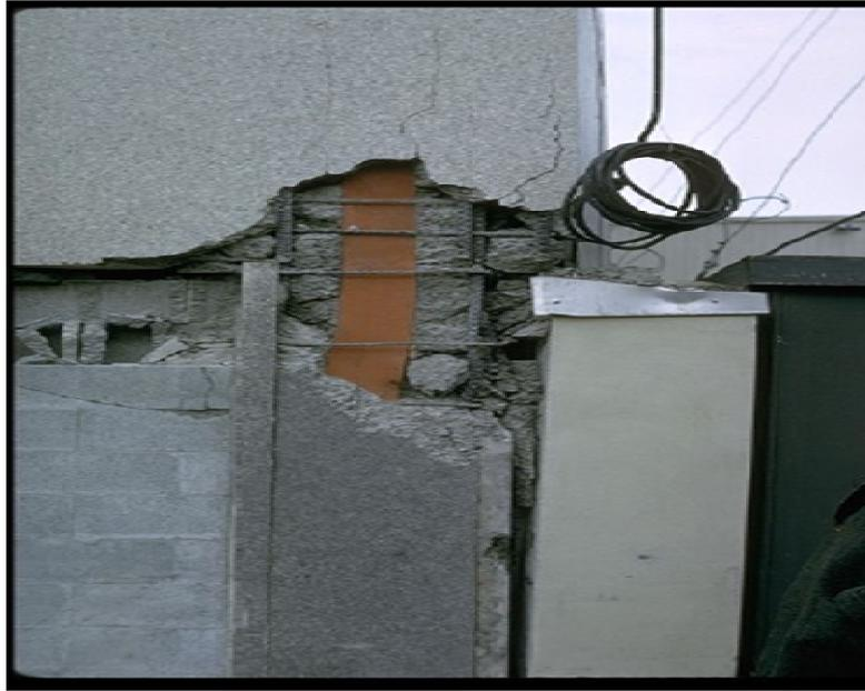
Figure 1.7. Joint parasismique insuffisant [19].
