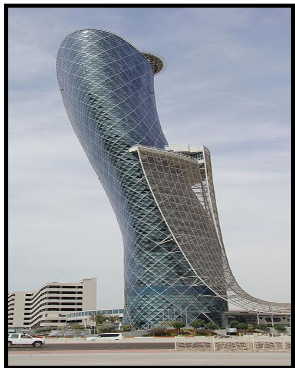
Fig. 49. La tour Capital Gate. Source : https://en.wikipedia.org/wiki/Capital_Gate
