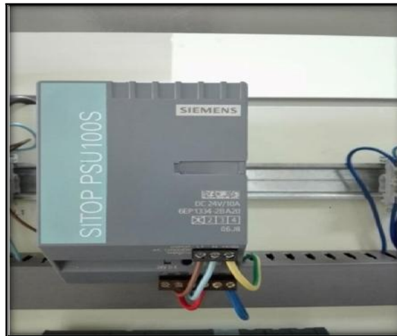
Figure 3.5: L'alimentation PSU100S
