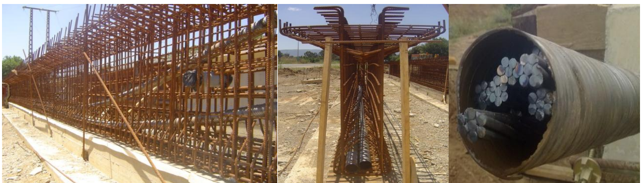
Figure XVII.13 ;14 ;15 :armatures passif et active
