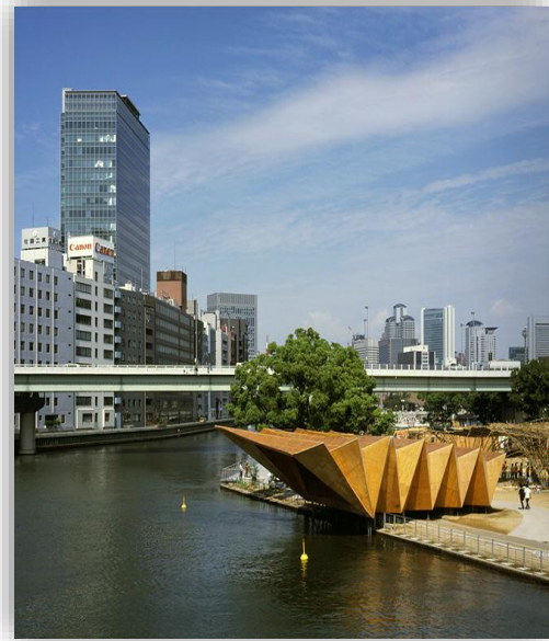
Figure 63: Aqua Metropolis pavillon
