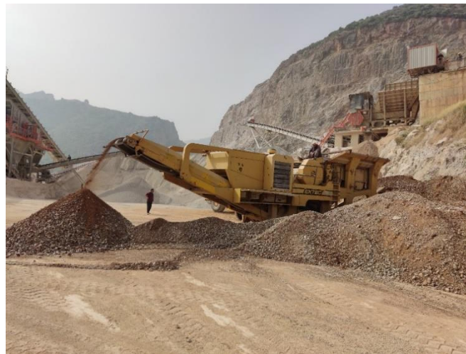
Figure 16: Station de concassage mobile.
