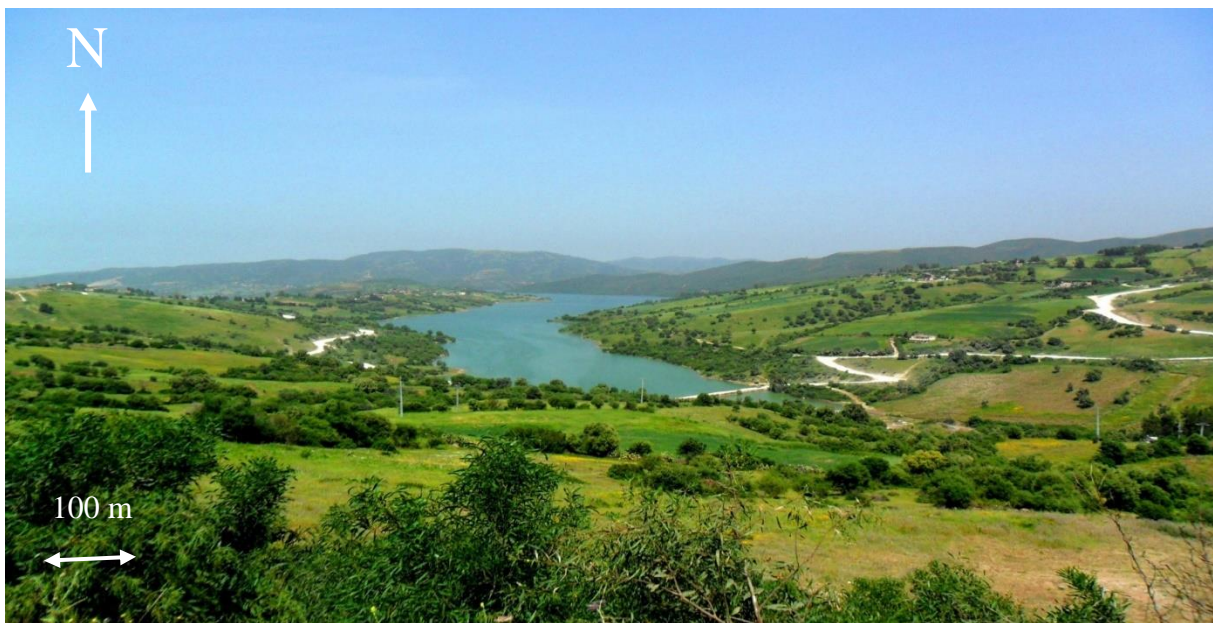
Figure 29: Barrage de Keddara.
