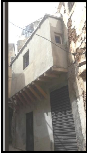
Figure 2: transformation de façades
