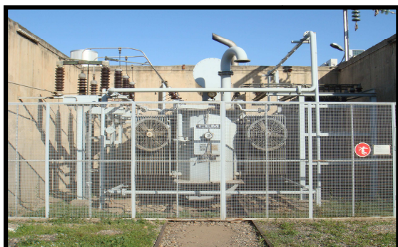
Figure I.10: Transformateur 11.5/63kV Figure I.11: Transformateur 11.5kV/400V
