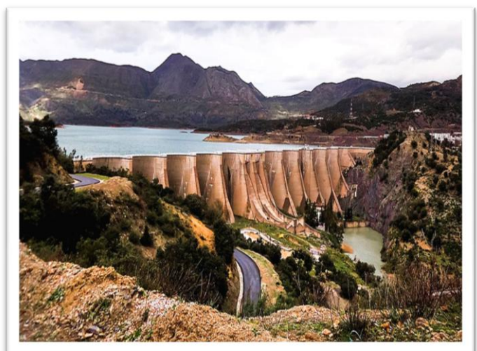
Figure 1.3 : Barrage Erraguene (Djijel).
