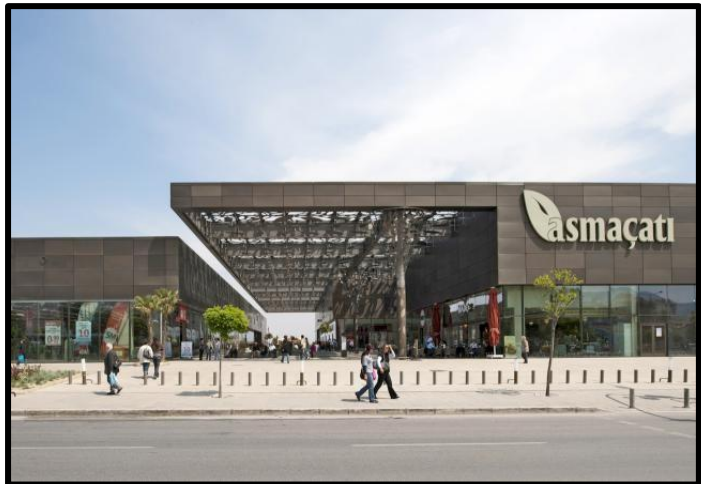
Figure 45: Vue globale du centre commercial Asmacati Source : https://www.archdaily.com/
