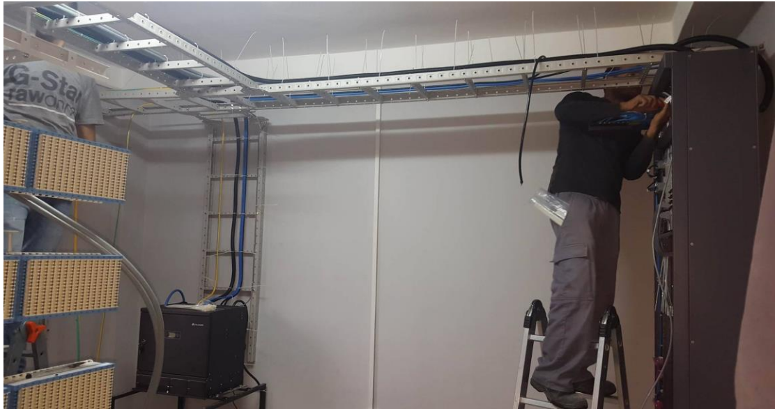
Figure III.19 : Raccordement des câbles.
