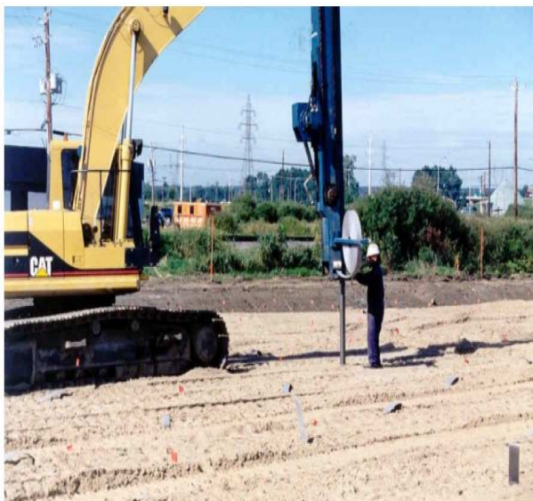
Figure II.15: Installation des drains verticaux
