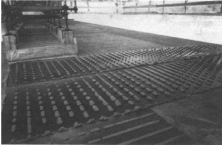
Figure I.13 plaques d'acier collées [5]
