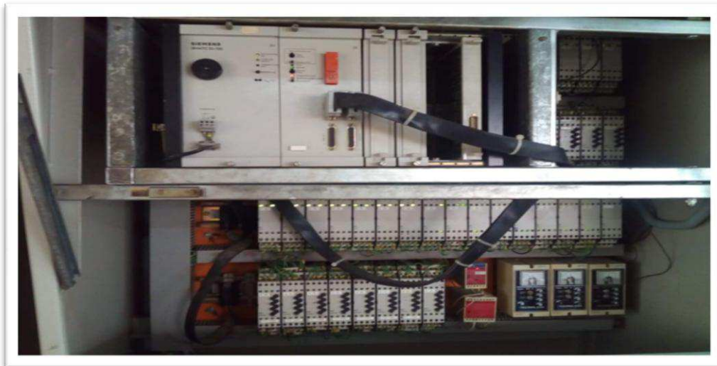
Figure III.2 : AUTOMATE S5-110.
