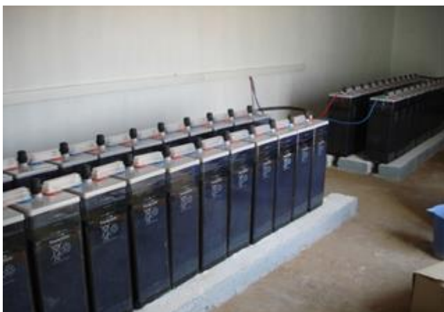
Figure 18 : Batteries solaires AGM
