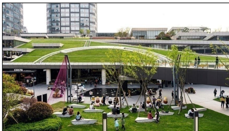
Figure 17: Groenland Center, Shanghai 2017.
