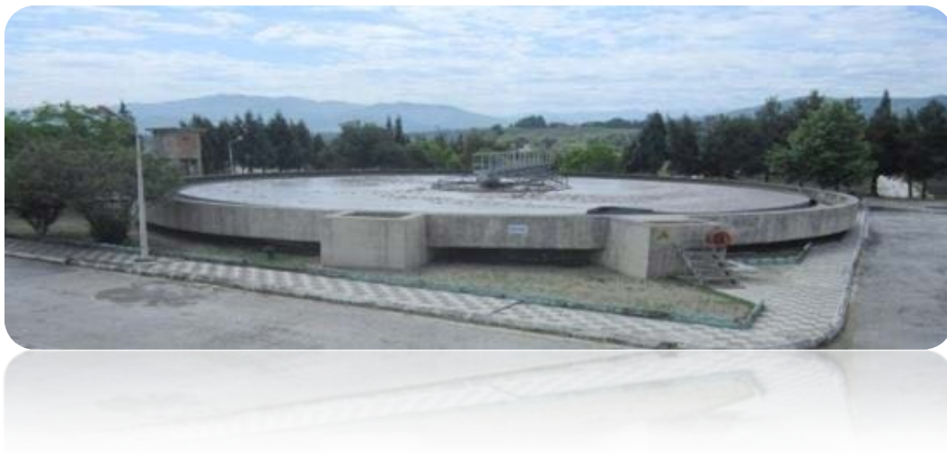
Figure II.6 : Clarificateur (ONA. Tizi-Ouzou, 2013)
