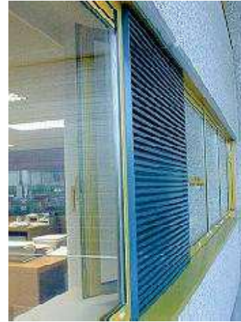
Figure I.24 : Grille de ventilation nocturne intensive
