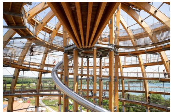
Figure 93:Sphère en bois Steinberg am See source:archdaily.com
