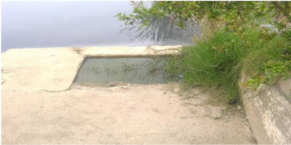
Figure 15: Station 1 ou le Gite 1 Station de pompage
