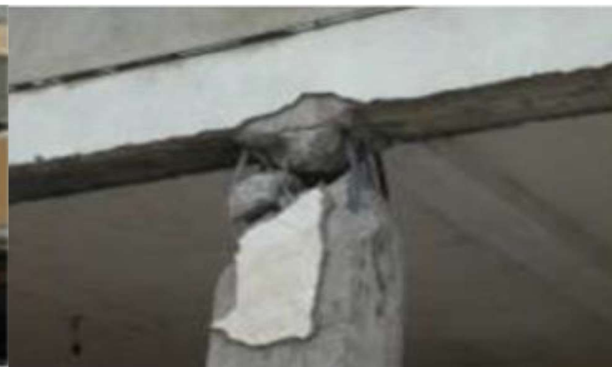
Figure I. 21: Dislocation de la section [18].
