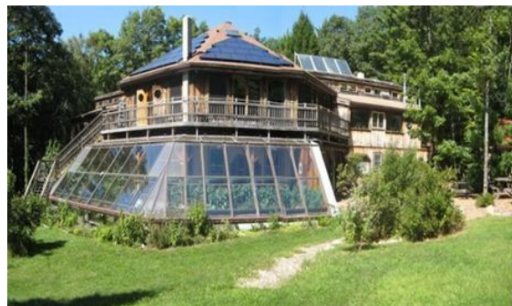
Figure 57 : Sirius Community Source : Build-Green.fr
