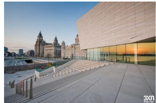
Fig 111 facade Source : www.archdaily.com/
