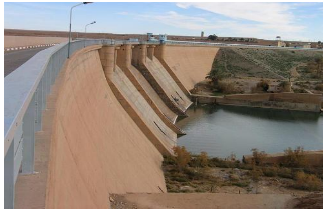
Figure 1.17 : Barrage DJORF TORBA [17]
