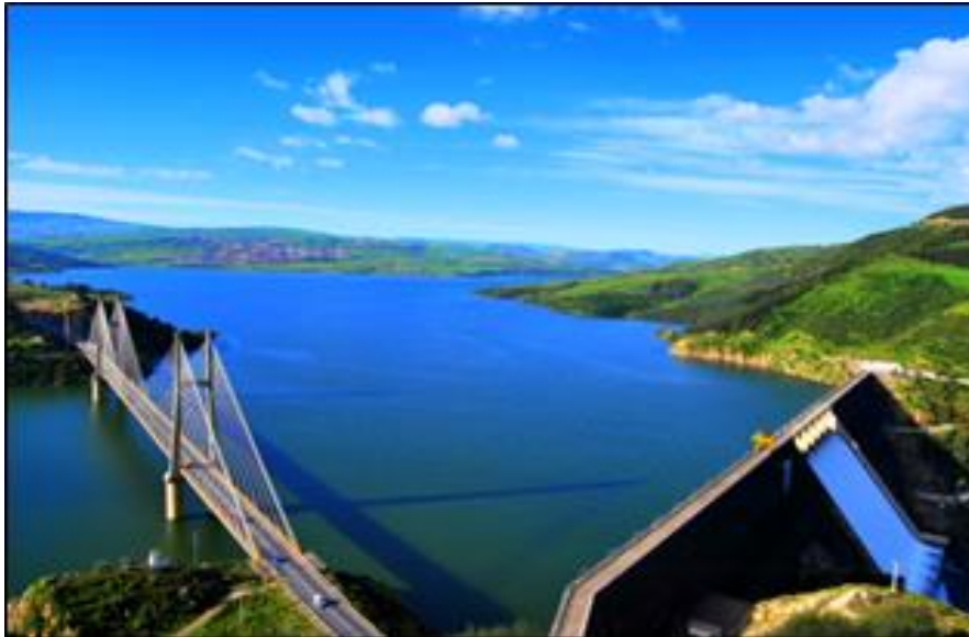
Figure 1.15 : Barrage BENI HAROUN [15]
