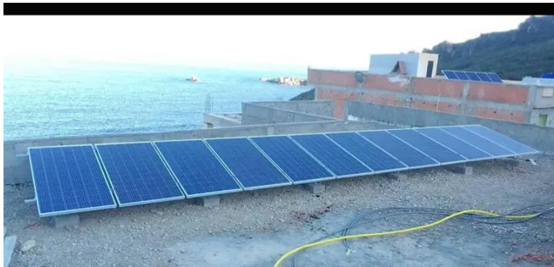
Figure 29: Installation panneaux Solaire
