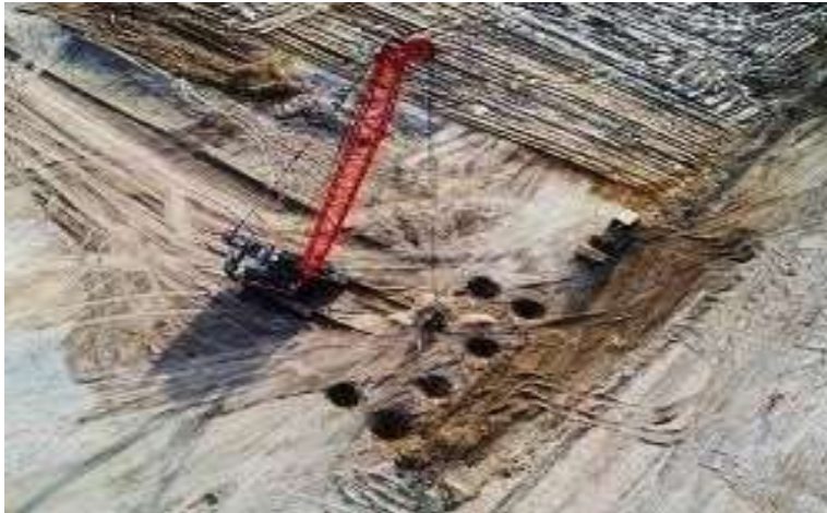
Figure II.1. Compactage dynamique.
