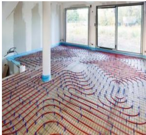
Figure I-64 : plancher chauffant rafraichissant.
