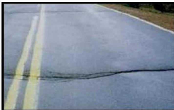
Figure III.20: Fissure transversale.
