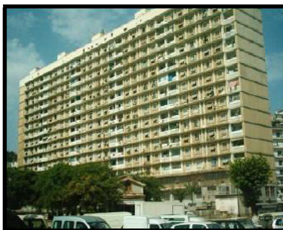
Figure 39: Bâtiment type H.B.M Source : https://www.google.com/search?q=batiments+hbm+hamma/
