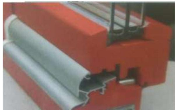
Figure 208:Triple vitrage
