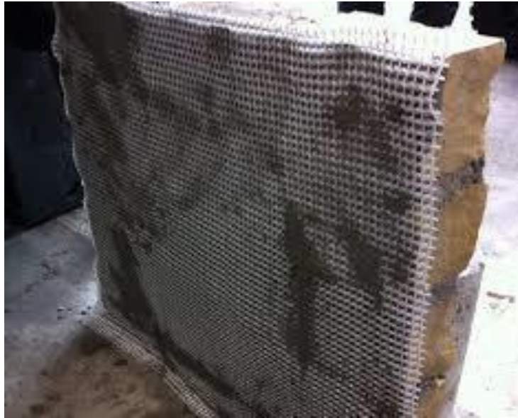
Figure III.17: Renforcement des murs [11].
