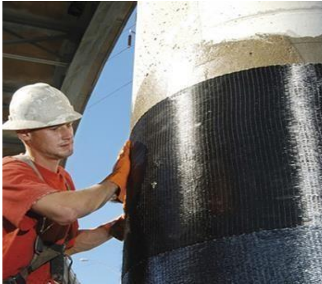
Figure III.14: renforcement des poteaux. [10].
