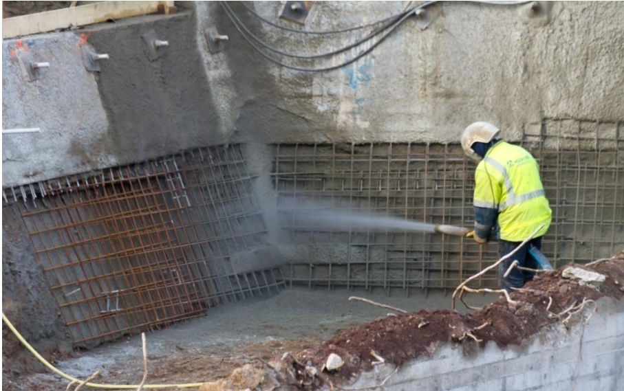
Figure I.6 : Projection du béton [26]
