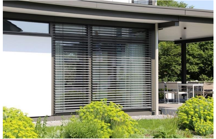
Figure 14 : brise soleil verticale
