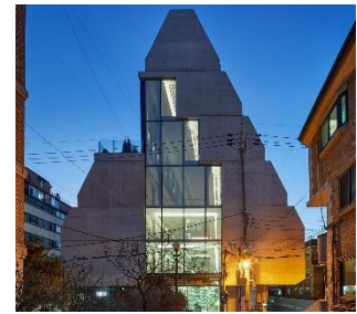
Figure 61 : Tree house Co-living(1), Source : www.archdaily.com
