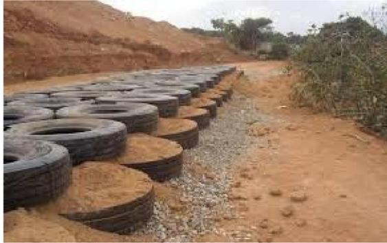
**Figure III-17 technique pneu sol**
