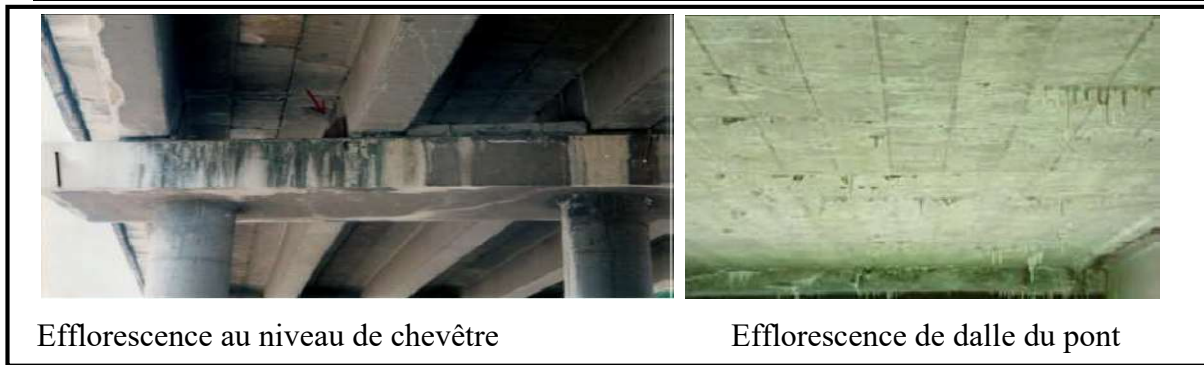
Figure I.7 : Efflorescence
