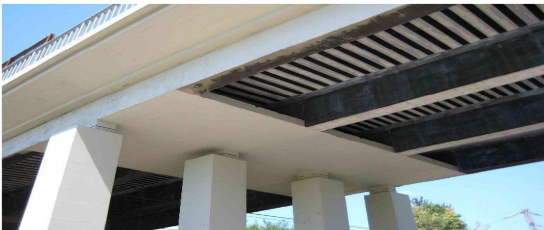
Figure II.8 : Renforcement des dalles.
