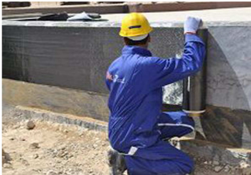
Figure II.9 : Renforcement des dalles
