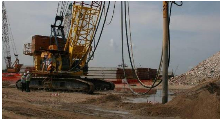
Figure 2.16. Vibrocompactage.
