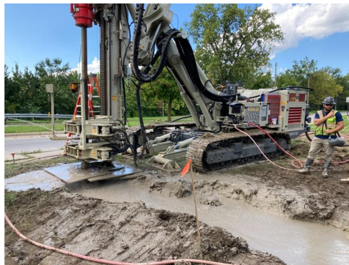
Figure 3.7. Technique de jet grouting.
