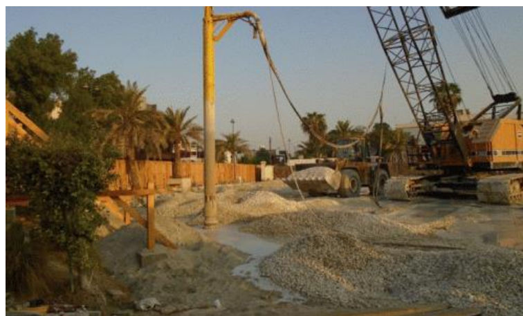
Figure 2.17. Vibro-remplacement.
