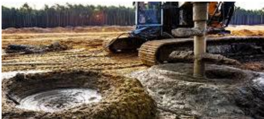
Figure 3.9. Technique de soil mixing.
