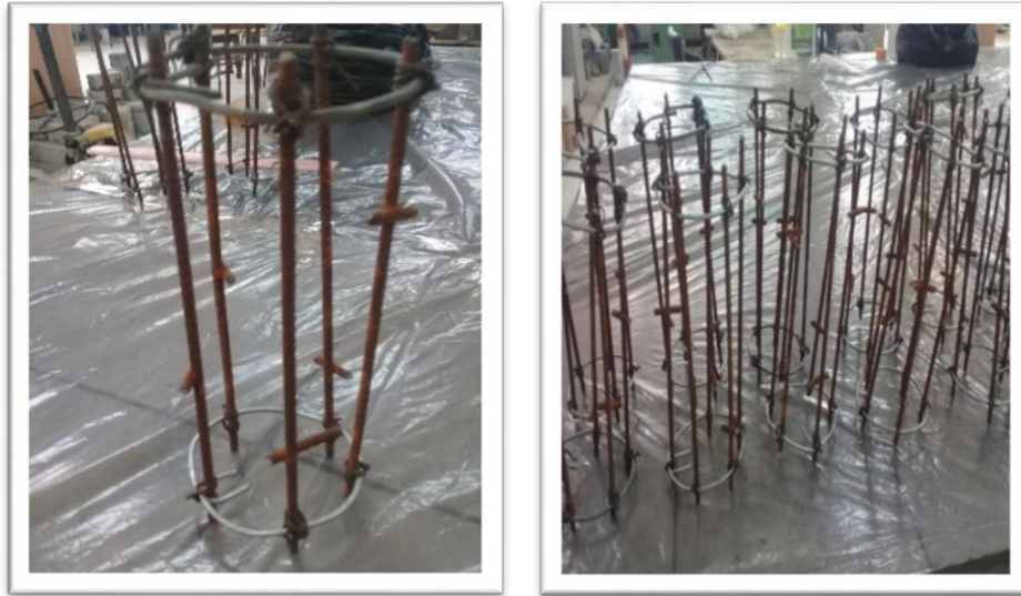
Figure 28: Ferrailage cylindrique[44].
