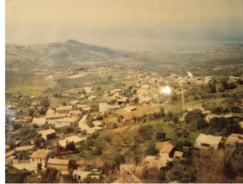
Figure 2: ancienne photo du village Source : E.R 22/12/2022
