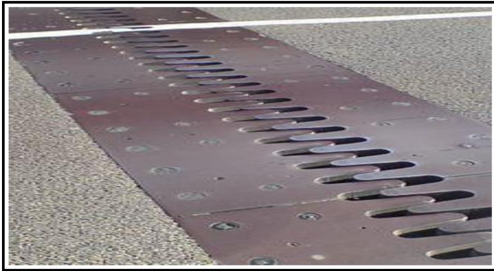
fig.-7 Joint de chaussée
